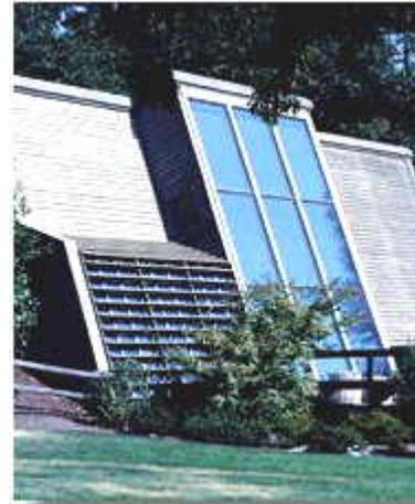
Water is pumped through pipes in the panel. The pipes are painted black, so they get hot when the Sun shines on them.
