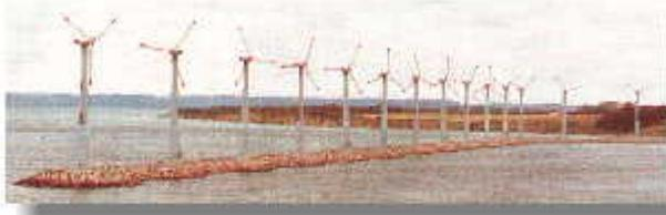
The propellers are large, to extract energy from the largest possible volume of air. The blades can be angled to "fine" or "coarse" pitch, to cope with varying wind speeds, and the generator and propeller can turn to face the wind wherever it comes from.
